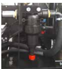
Direct water pumping system with self-cleaning filter and antiscaling pump
